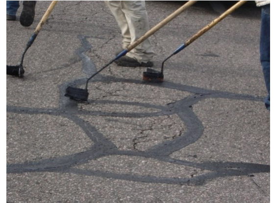
Crack Sealing/Filling
