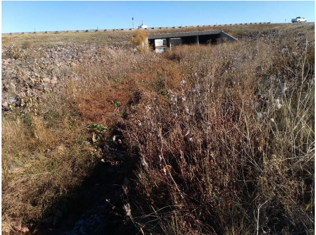
Photo 5. WL-1 west of West Cargo Road along Third Creek, facing east.
