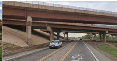
Existing condition: CO 224 under I-270
