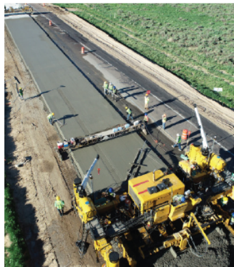
Construction on US 287 in Larimer
