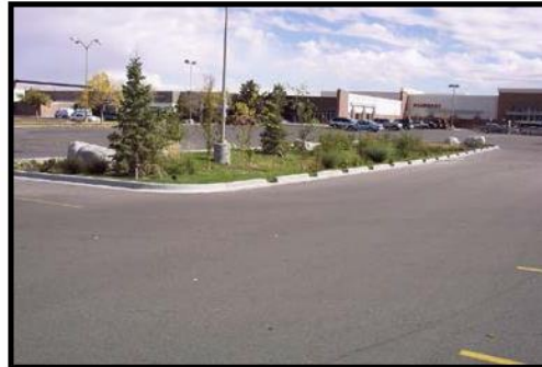
Figure VII-3. Examples of Curb Breaks for Stormwater Runoff
