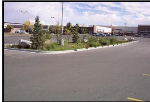
Figure VII-3. Examples of Curb Breaks for Stormwater Runoff
