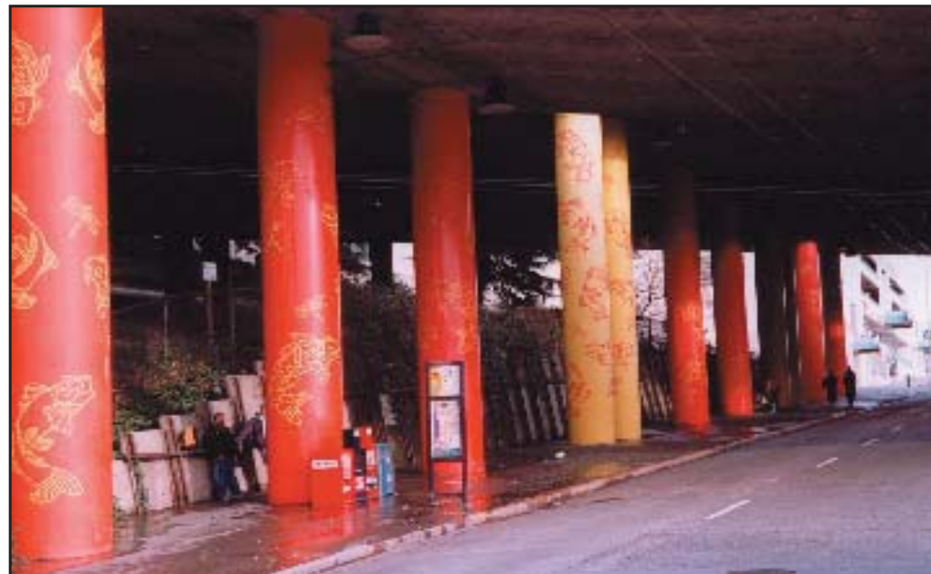
Painted colonnades underneath the I-5 freeway
