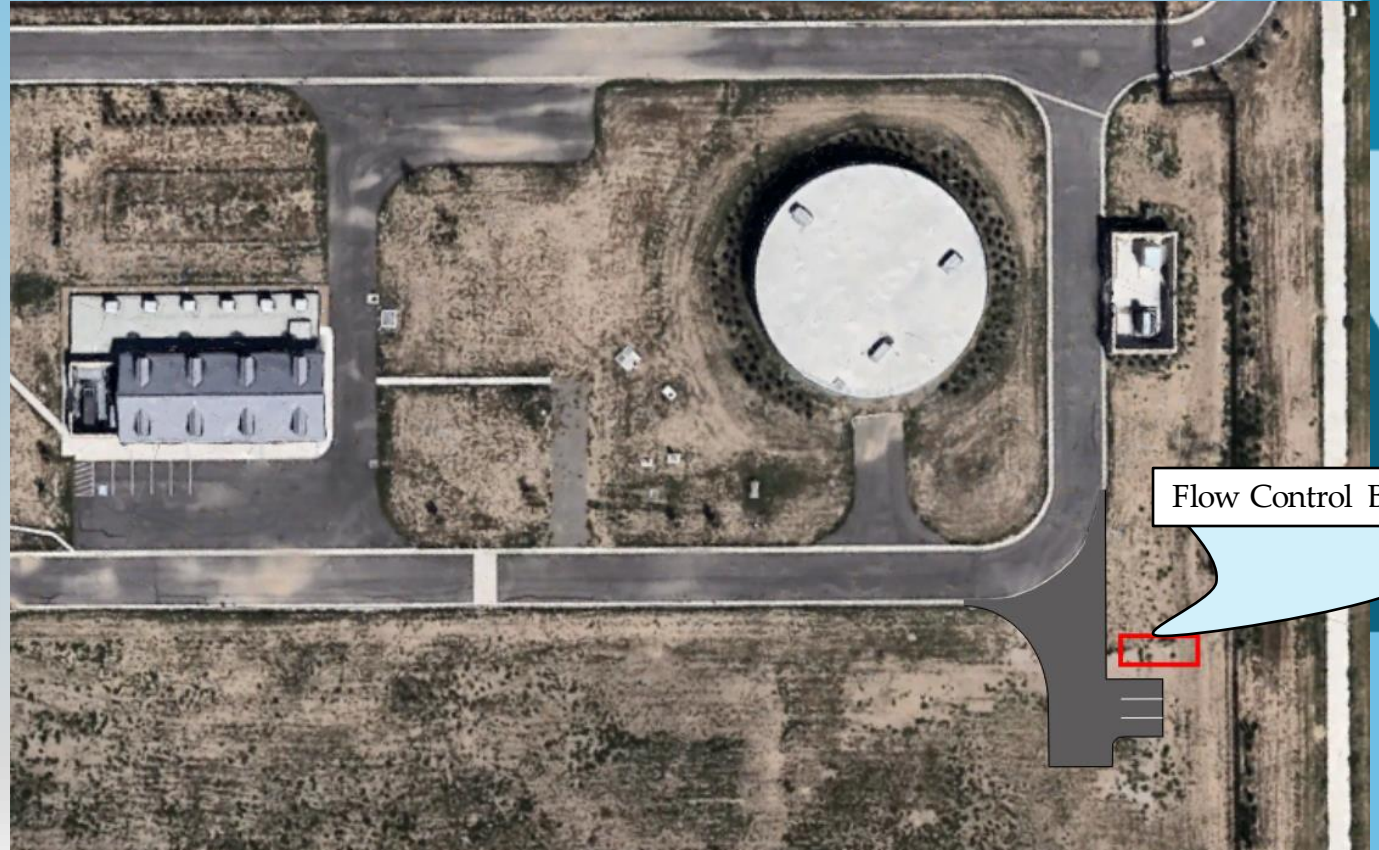
Prairie Waters Pump Station No. 2
